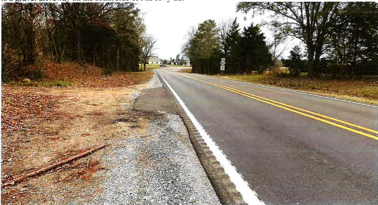
Above: MS Hwy 22 looking west at existing gravel drive/proposed site driveway.
