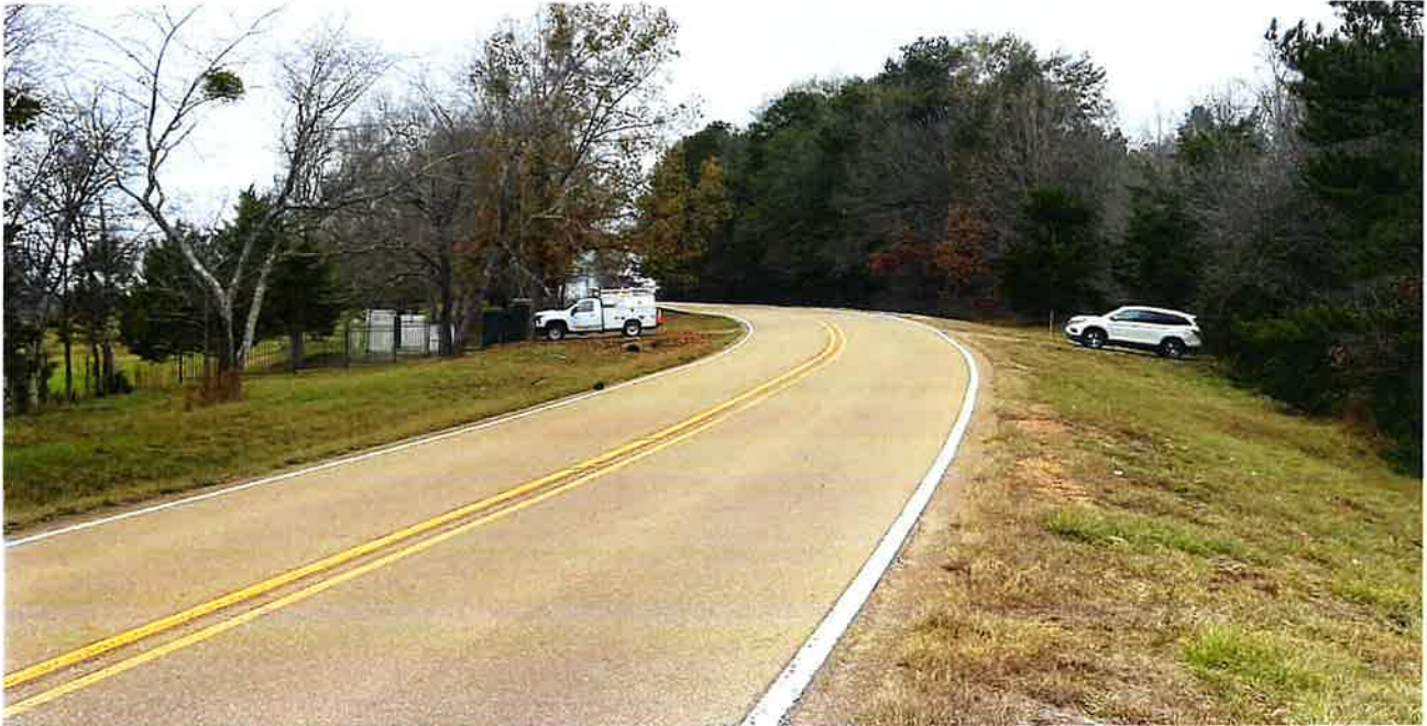
Above: MS Hwy 463 looking north. Vehicle on right in existing gravel driveway. Vehicle on left at utility drive.
