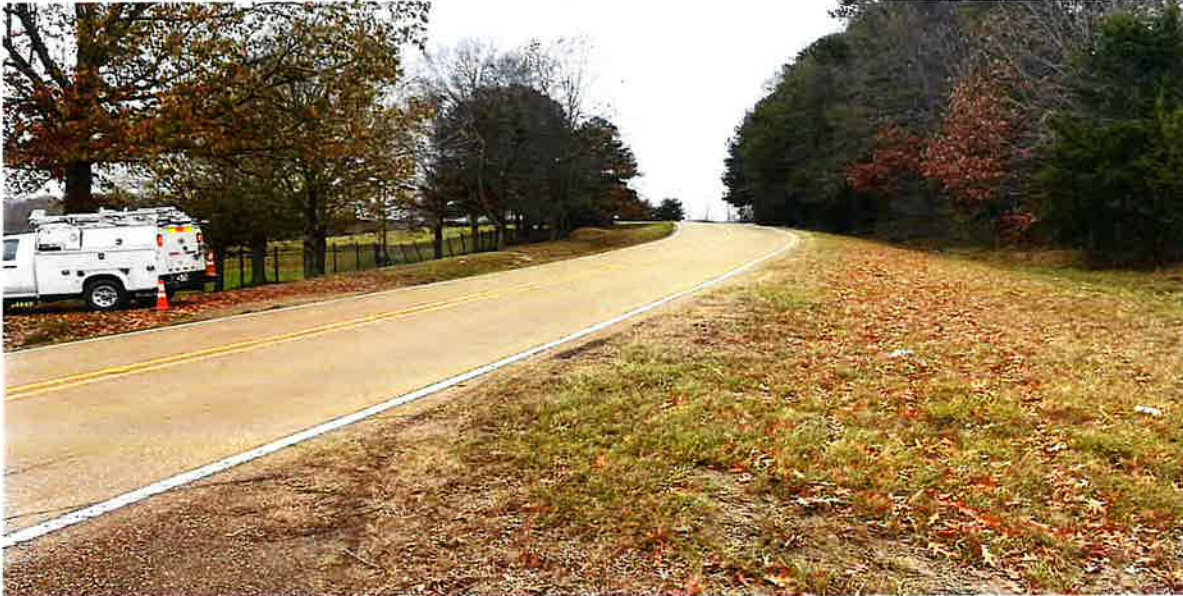
Above: Looking north along MS Hwy 463 toward Chestnut Hill driveway.
