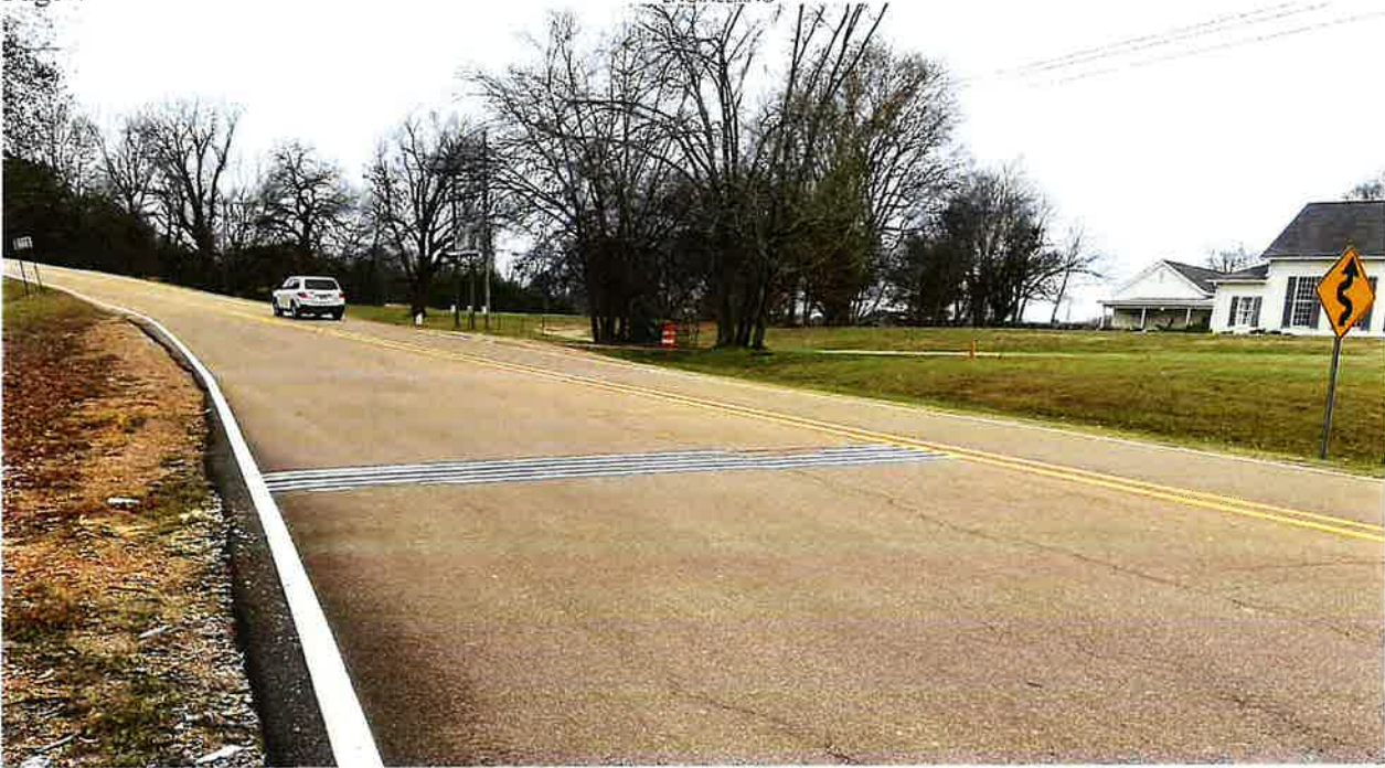
Above: Looking south on MS Hwy 463 at rumble strips and gated driveway to Livingston church.
