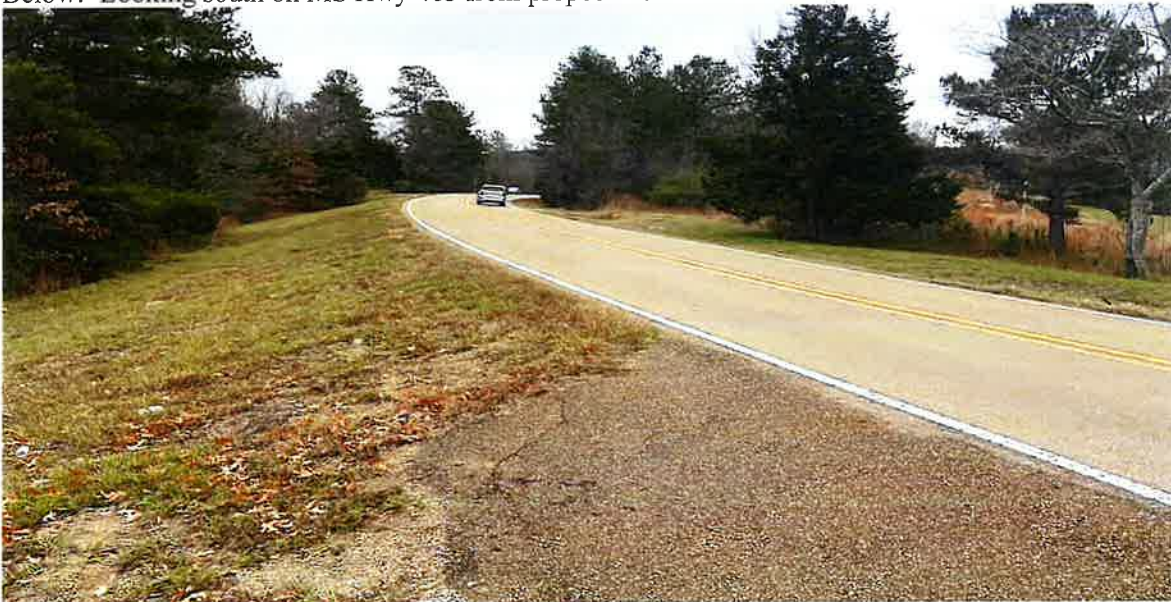
Below: Looking south on MS Hwy 463 from proposed South Site Drive.
